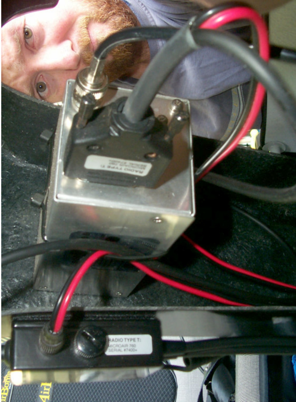
PHOTO SHOWS WIRE ROUTING AFTER INSTALL.
